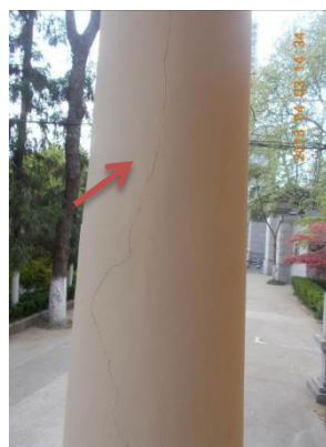
砖柱竖向裂缝
