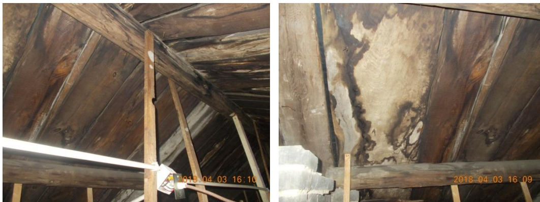
木构件老化、渗水腐朽
